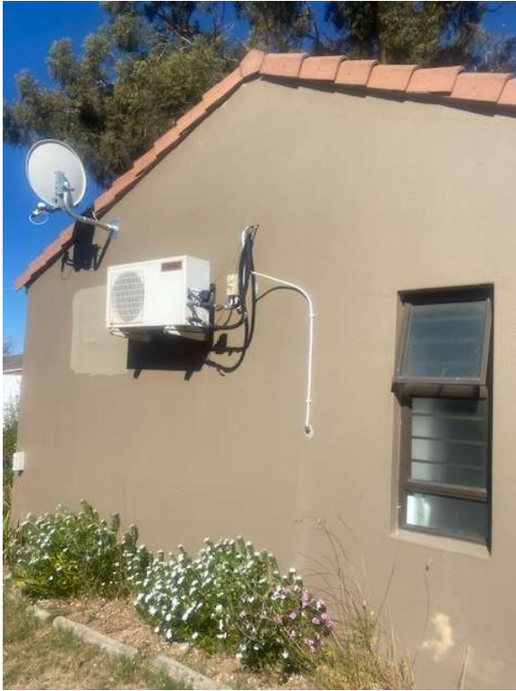
Figure 3 - Localized plaster damage and cracking at low level due to slab movement.
