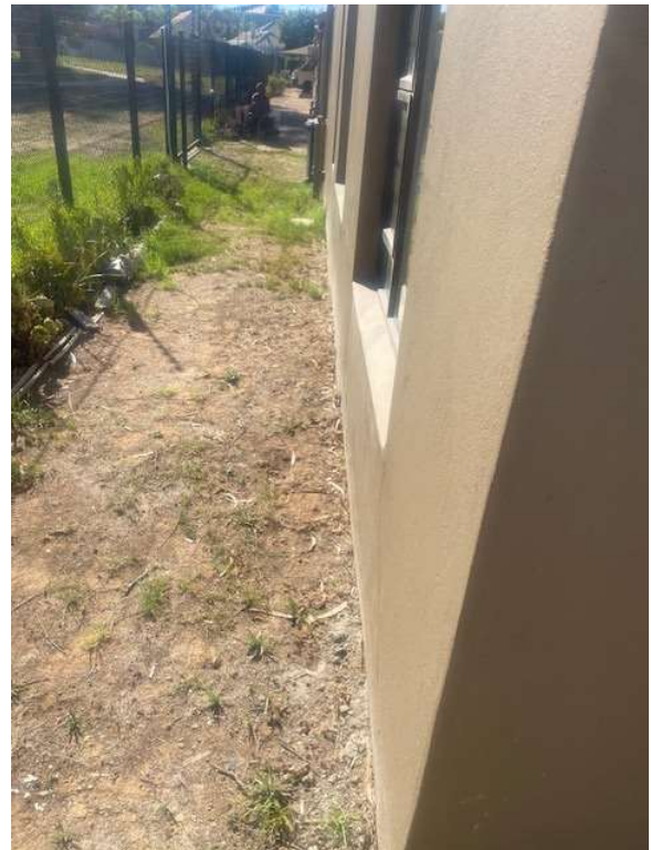
Figure 8 - Wall-to-floor junction failure showing detachment of finishes due to movement.
